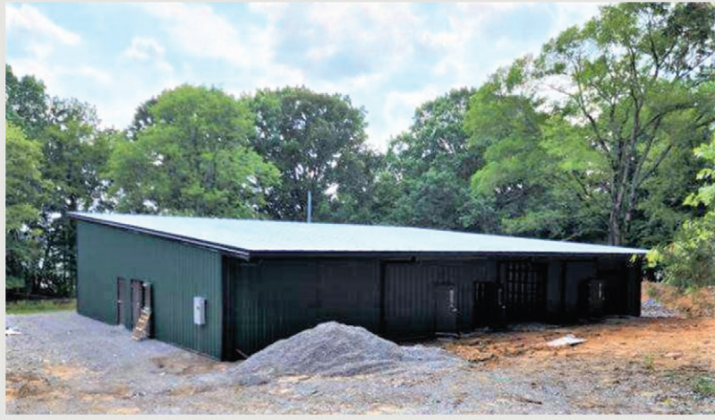
As of July 12, 2022 the building was in place
