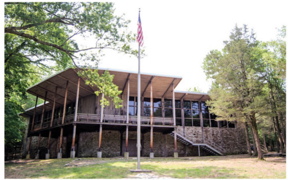
Camp Craig Dining Hall Renovation
