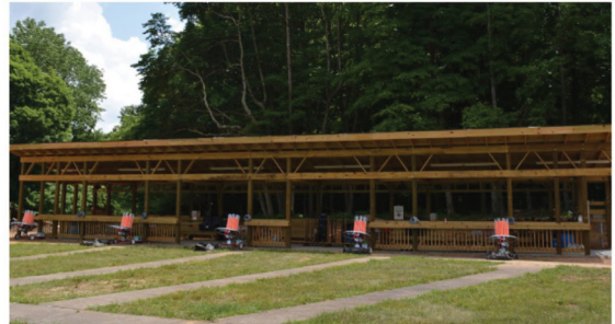
Menefee Shotgun Range Renovation
